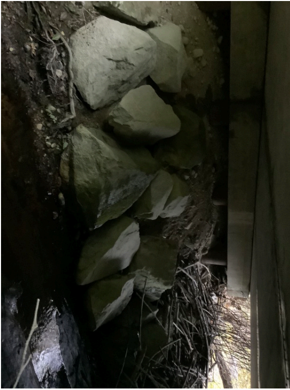
Right Bank Abutment when facing downstream
