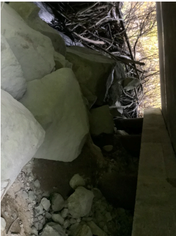
Left Bank Abutment when facing downstream
